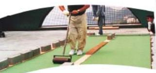
Start work on one side of the court and stop near the middle. The last roll at the middle of the court is only adhered along half its width. Then start work from the opposite side and do the same. Always weight down seams and always roll the surface. Monitor your glue consumption.
