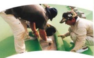
The two rolls in the middle of the court are opened. Adhesive is applied by trowel or brush and the seams carefully closed. Remember to weight the seams and to continue rolling the surface until the adhesive has set.
