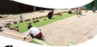
Once the adhesive has partially set, use a hand held roller to press the Decoflex material into the adhesive. The adhesive is still tacky enough to 'grab' the roll material. Rolling is done to ensure a complete bond to the base as well as eliminate possible air entrapment.
