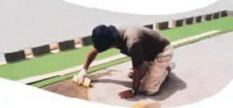
Once the adhesive has gone tacky, roll the Decoflex material into the glue, carefully following the seam of the preceding roll or snapped chalk line. Monitor your glue consumption.
