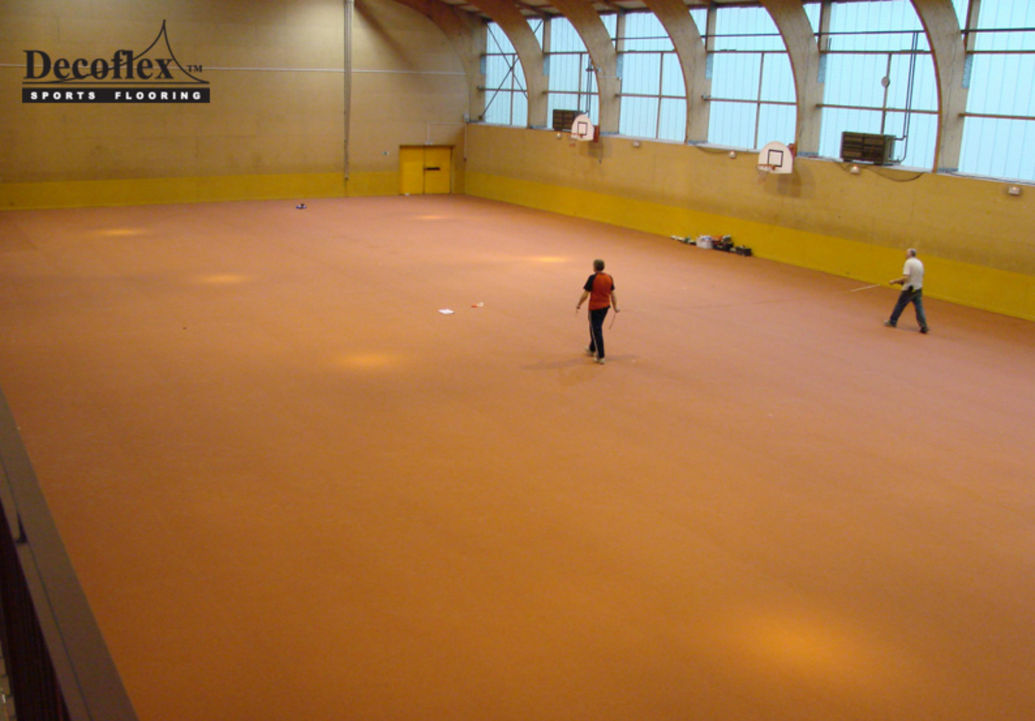
Decoflex 'D' Installation - EPDM Top Mat complete. Line Marking beginning.
